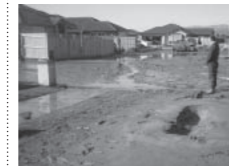
The liquefaction blocked whole streets in some areas of the city.
